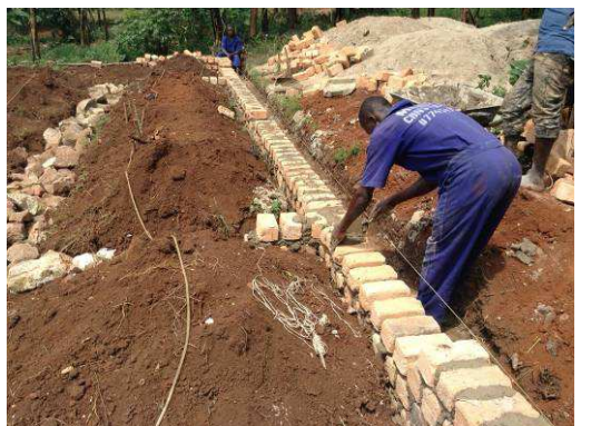
Laying the Foundations
