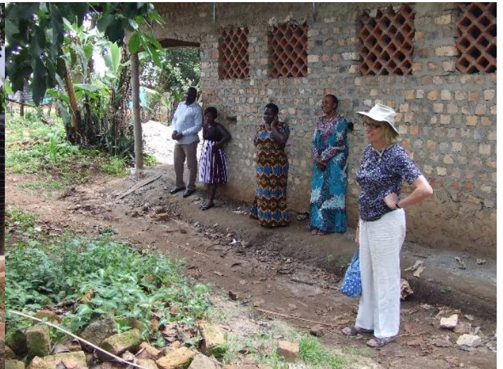
Rear wall which requires plastering. The apron needs to be completed
